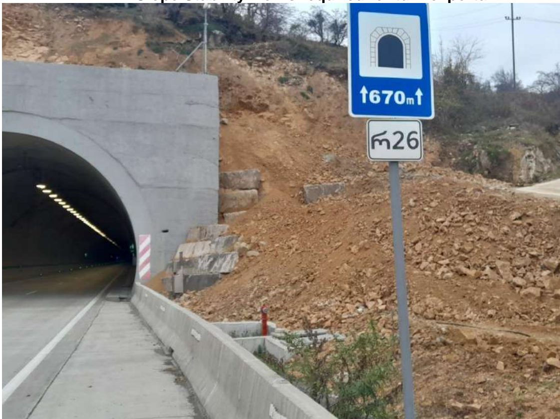
Slope Stability works required for tunnel portal
