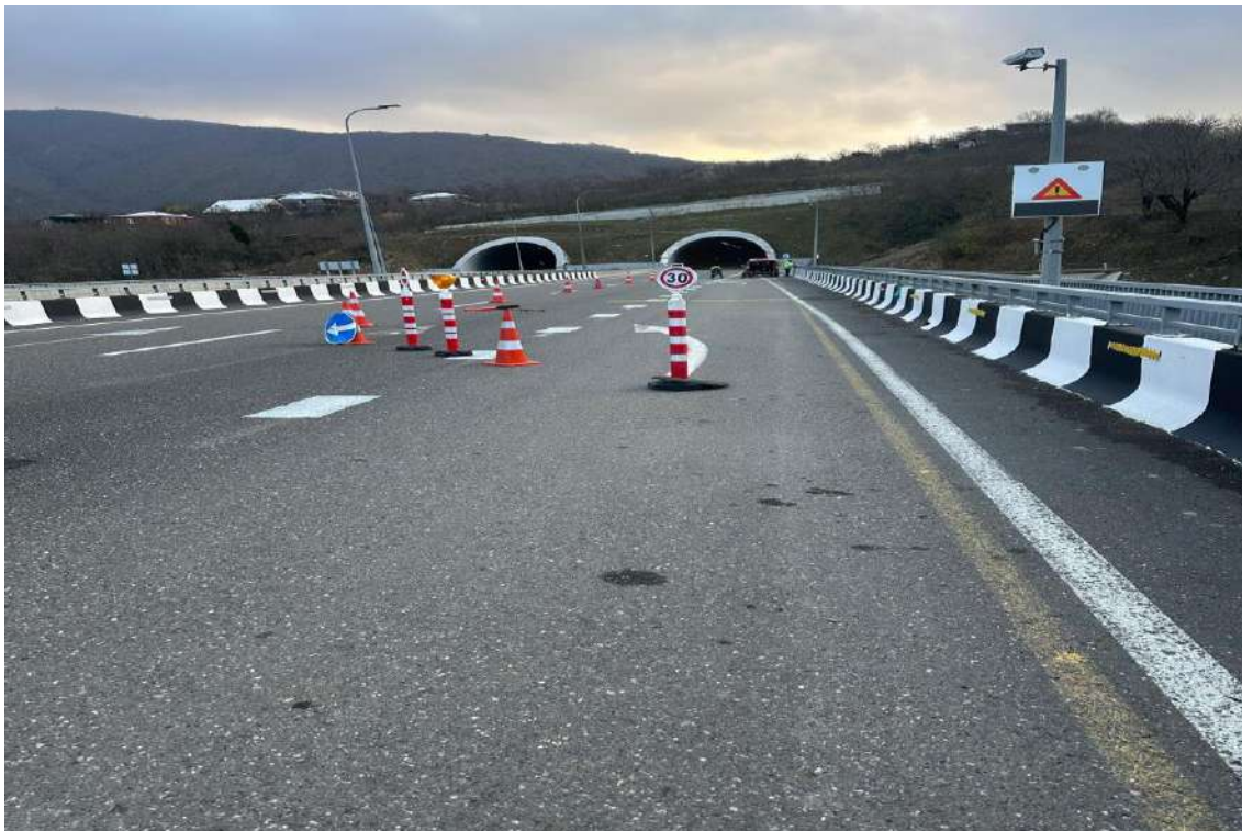
Figure 5: traffic diversion for road safety (November 2025)
