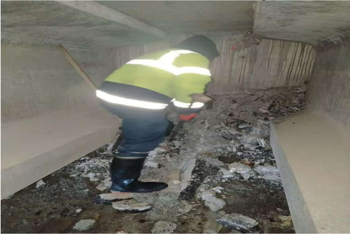
Maintenance works under the bridge
