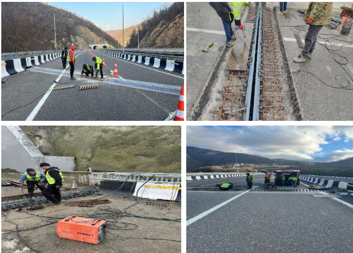
Figure 2: Ongoing maintenance works for bridges and tunnels during DNP (November 2025)
